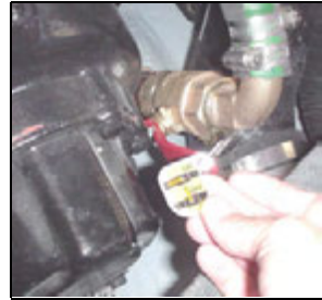
Engine Cooling Water Intake Shut-Off Valve
